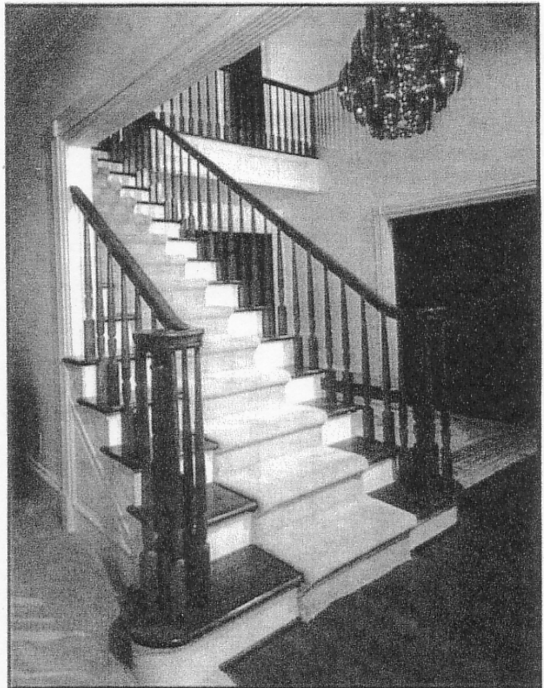
Pictured: S-6210 Handrail, F-3011 Volute Newels, F-3010 Starting Newel, F-2015 Balusters, S-7230 L.H. Volute, S-7235 R.H. Volute, S-8015 Starting Step.
